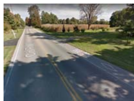
Figure 20E: Cleveland Road looking east
