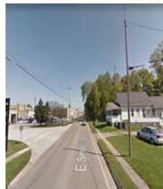
Figure 17F: Strub Road near the Ohio Veterans Home looking east
