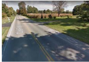
Figure 23E: Bogart Road looking east
