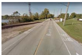
Figure 22E: River Road looking north
