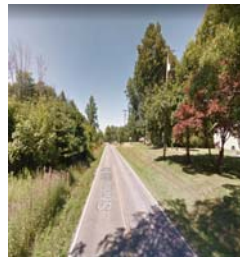
Figure 19F: Sunnyside Road looking north
