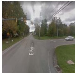
Figure 16F: Perkins Avenue and Strub Road looking southeast
