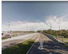
Figure 21E: Cleveland Road Bridge looking east
