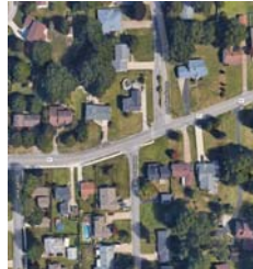
Figure 18F: Marshall Avenue looking north
